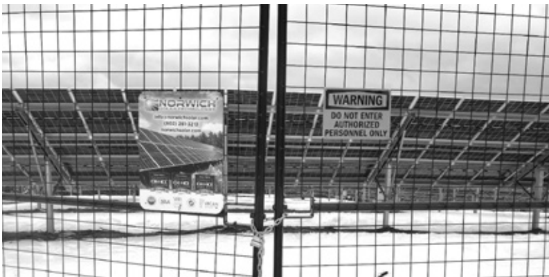
Center gate of 5-row western sub-array.
