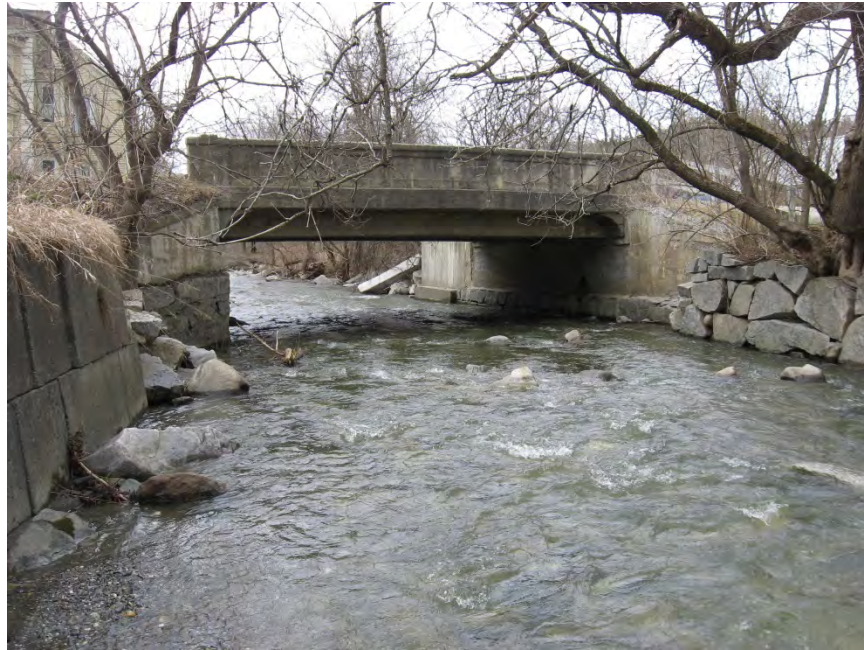
Figure 1: Mill Street Bridge Looking Downstream
