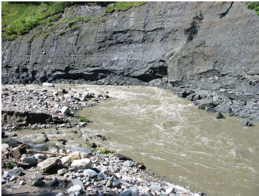
Figure 7: Landslide on Great Brook (Milone & MacBroom, Inc., 2015)
