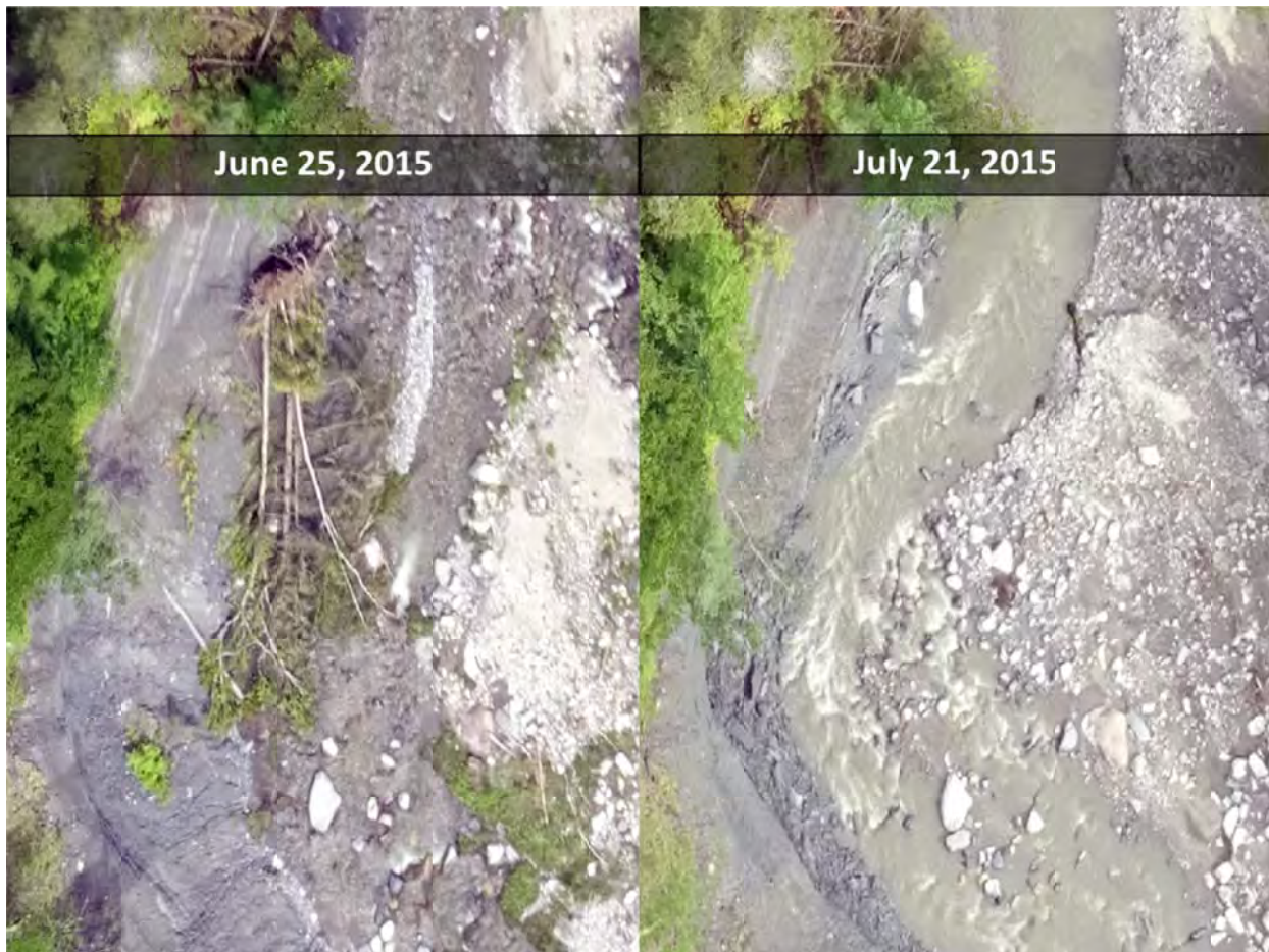
Figure 9: A Comparison of UAV Photographs Showing Wood Removal on Great Brook Approximately 300 feet Downstream of the Cameron Road Bridge (O’Neil-Dunne and Ahles, 2015)
