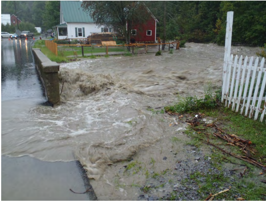
Figure 3: Upstream Face of the Brook Road Bridge Full (Springston, 2011)
