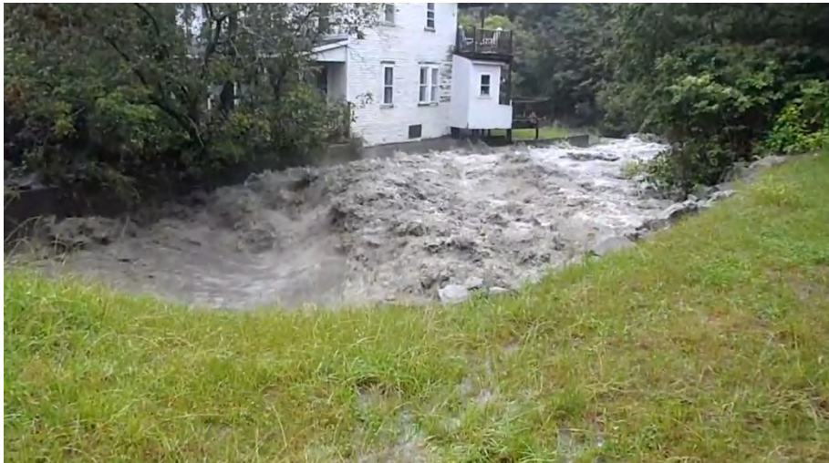
Figure 4: Hydraulic Roller Downstream of Brook Road Bridge (Springston, 2011)
