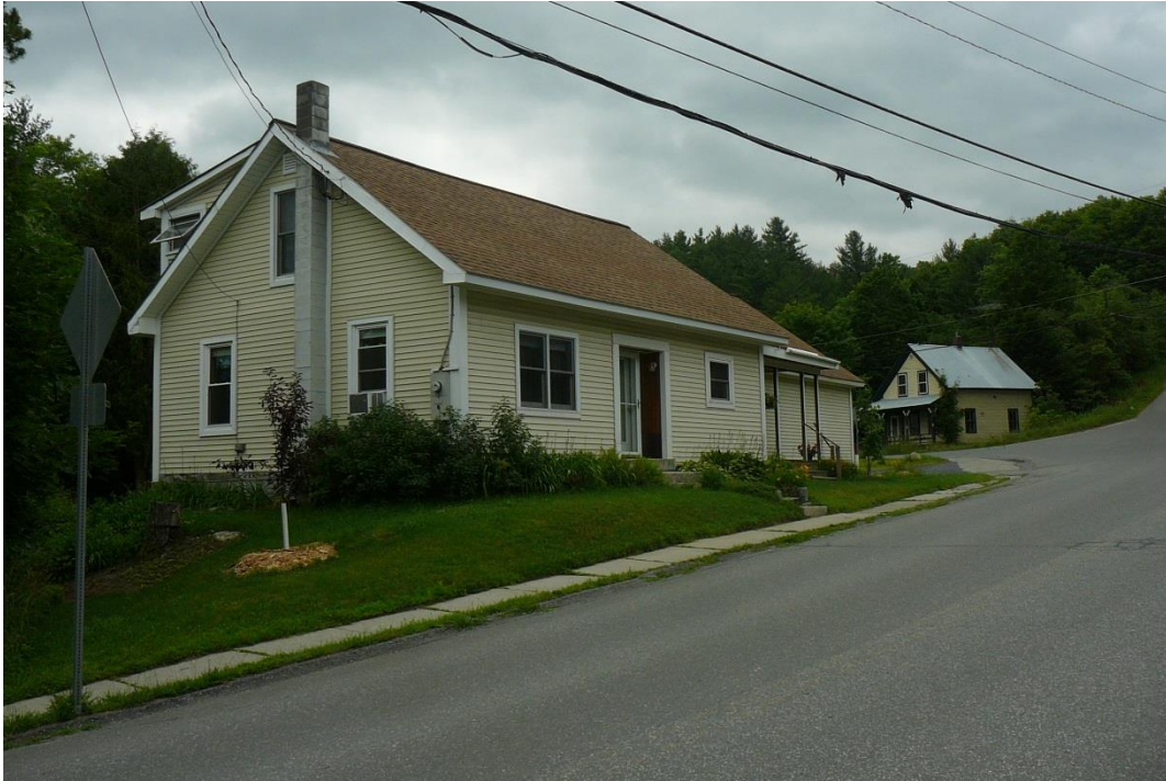
Figure 22. View southeast of 133 Mill Street.
