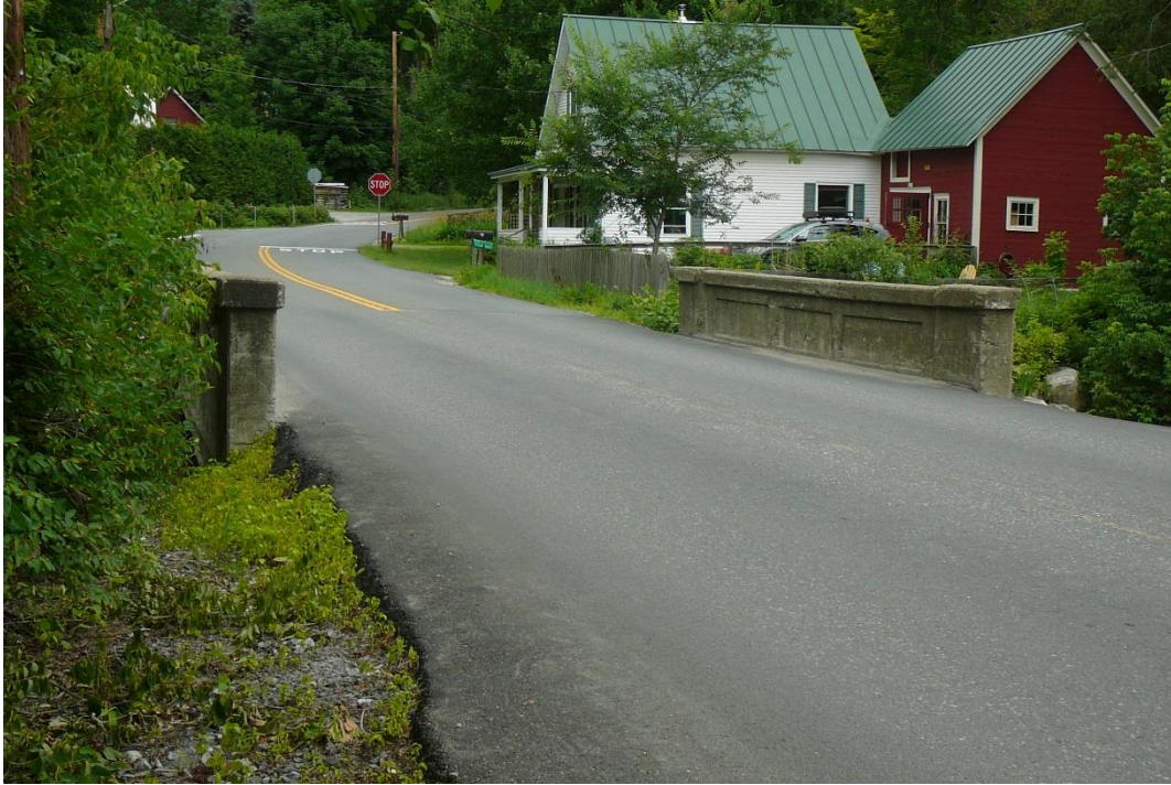
Figure 62. View southeast of Bridge 21 along Brook Road.
