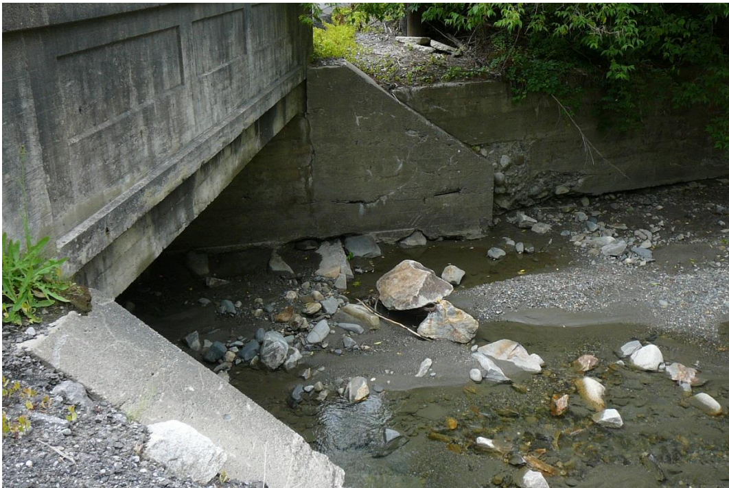
Figure 65. View west of Bridge 21 along Brook Road.
