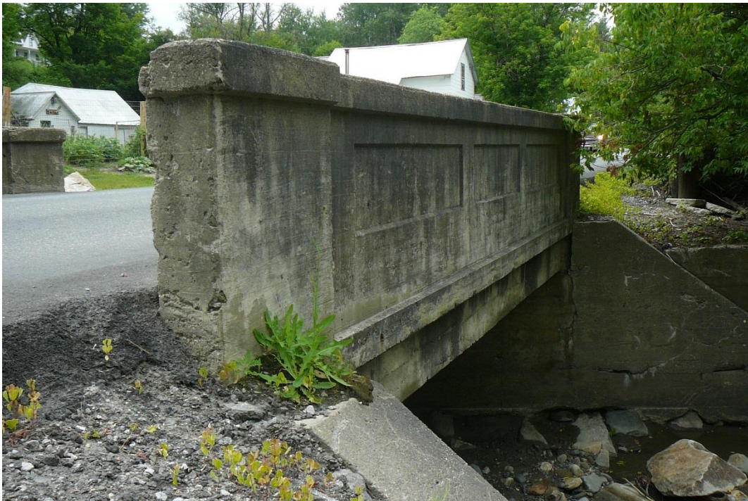
Figure 63. View west of Bridge 21 along Brook Road.
