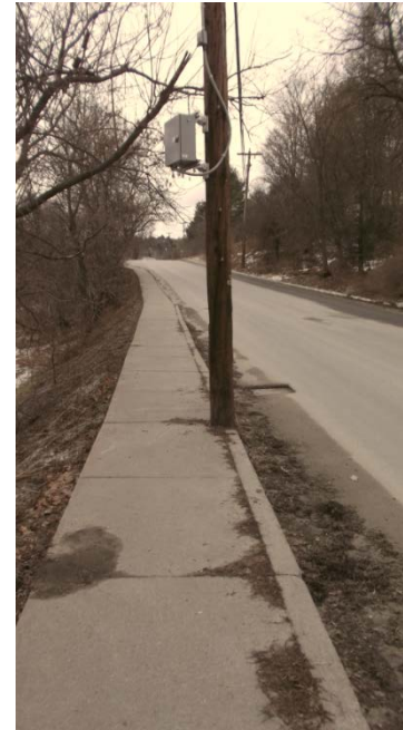
Image 4-7: Utility pole located on Main Street Sidewalk
