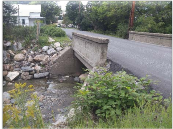
Image 4-4: Bridge on Brook Road
