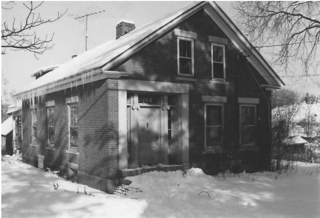
Figure 58. View northeast in 1981 of 191 Main Street.
