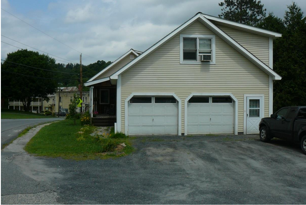
Figure 24. View north of garage at 133 Mill Street.
