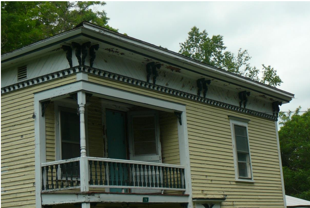
Figure 45. Close-up view of second story porch, stickwork frieze board and roof line brackets at 78 Creamery Street.
