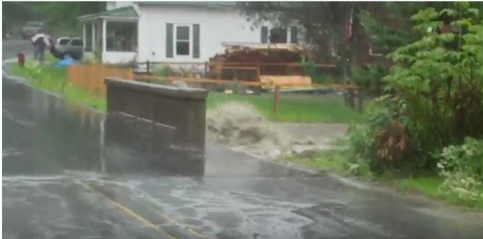
Figure 60. Clip from You Tube video showing flooding at Bridge 21 during Hurricane Irene at the end of August 2011 (You Tube September 2011).
