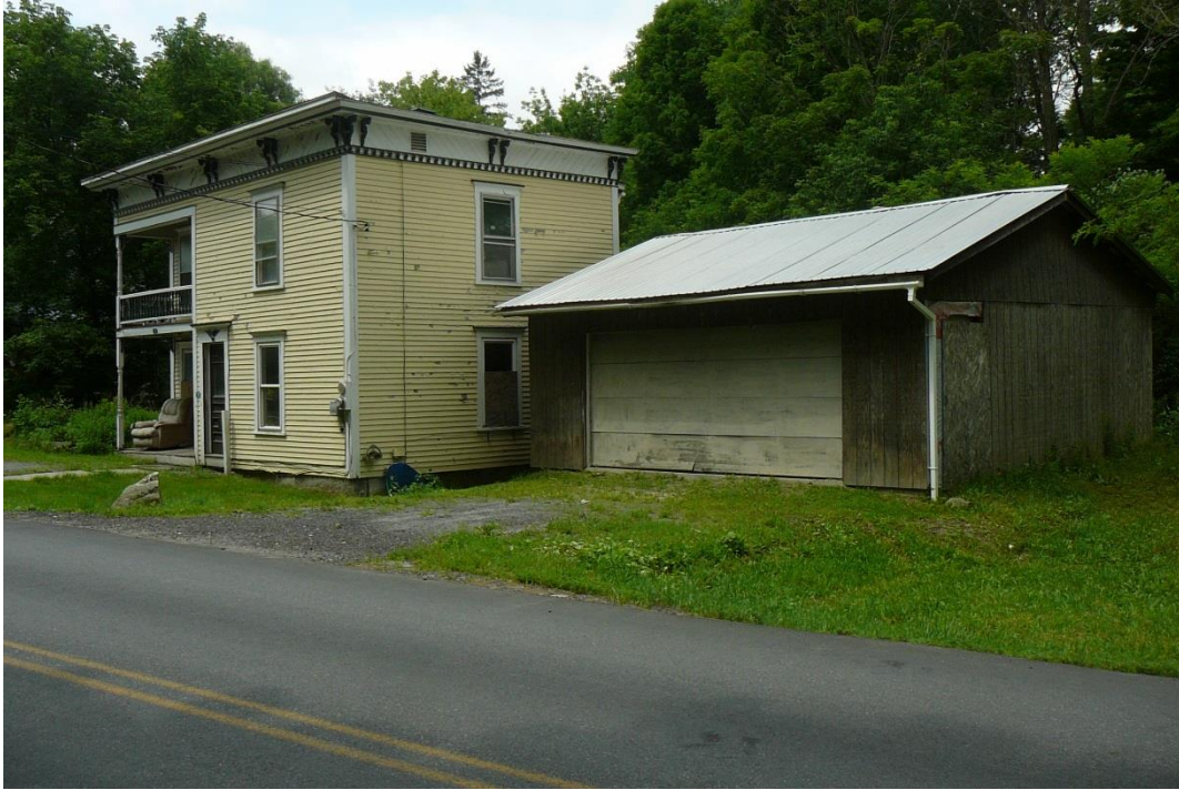
Figure 44. View southwest of 78 Creamery Street.
