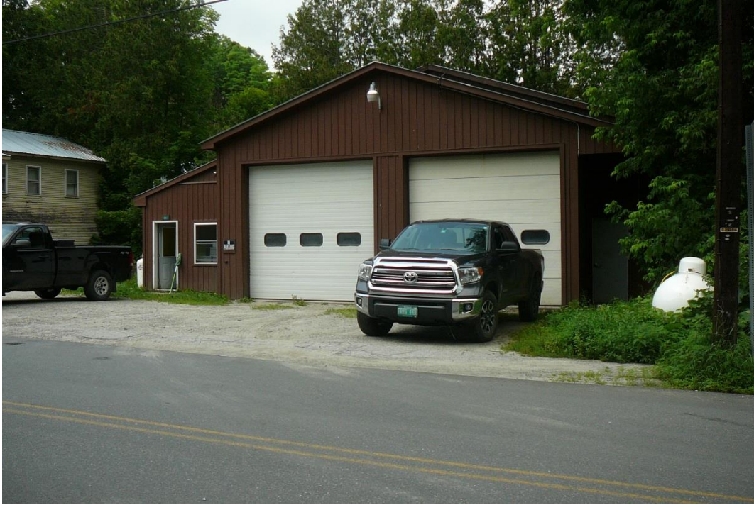
Figure 51. View southwest of 30 Creamery Street.
