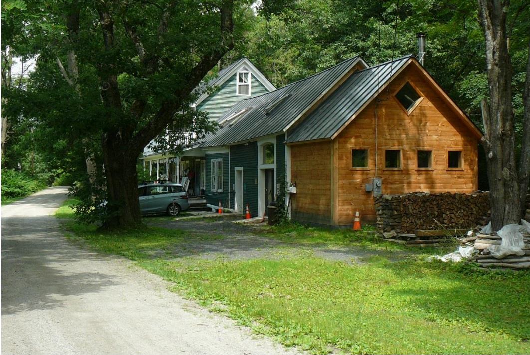
Figure 38. View northwest of 123 Hudson Avenue.
