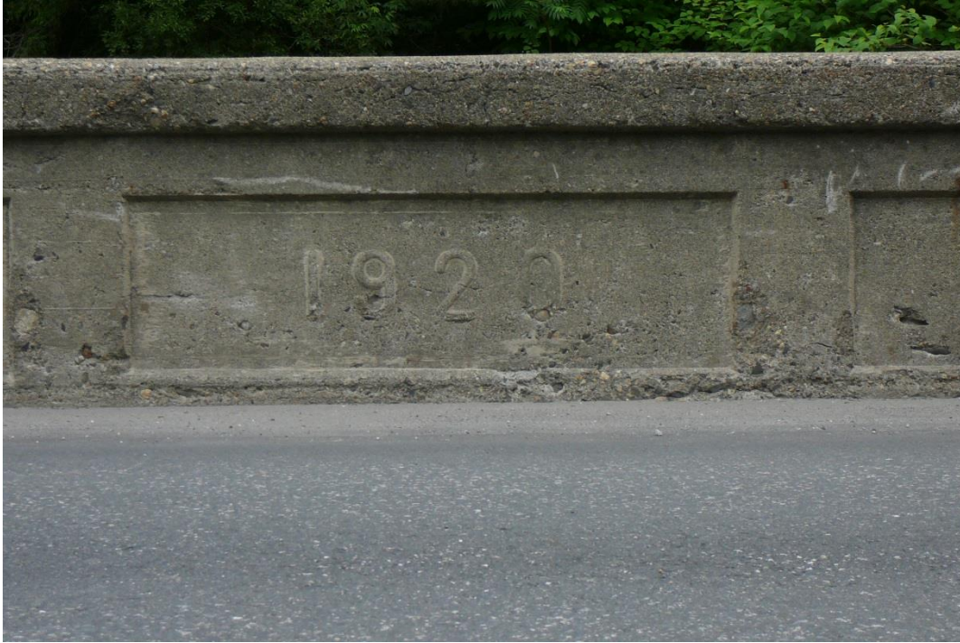
Figure 64. View south of Bridge 21 along Brook Road.
