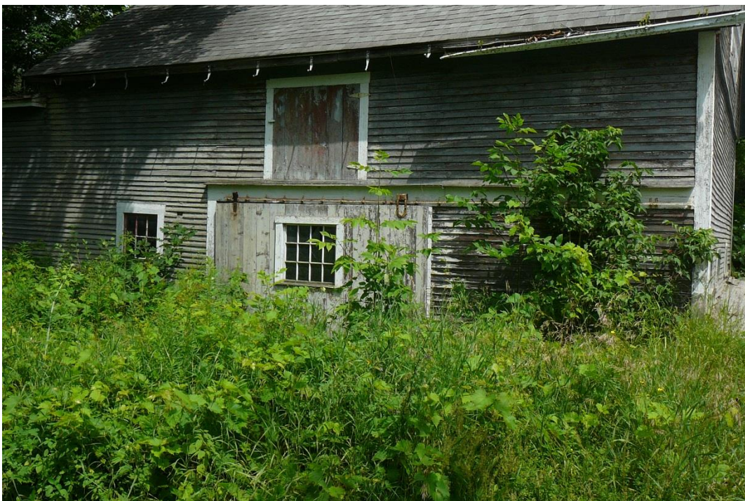
Figure 33. View northwest of barn at 99 Brook Road.
