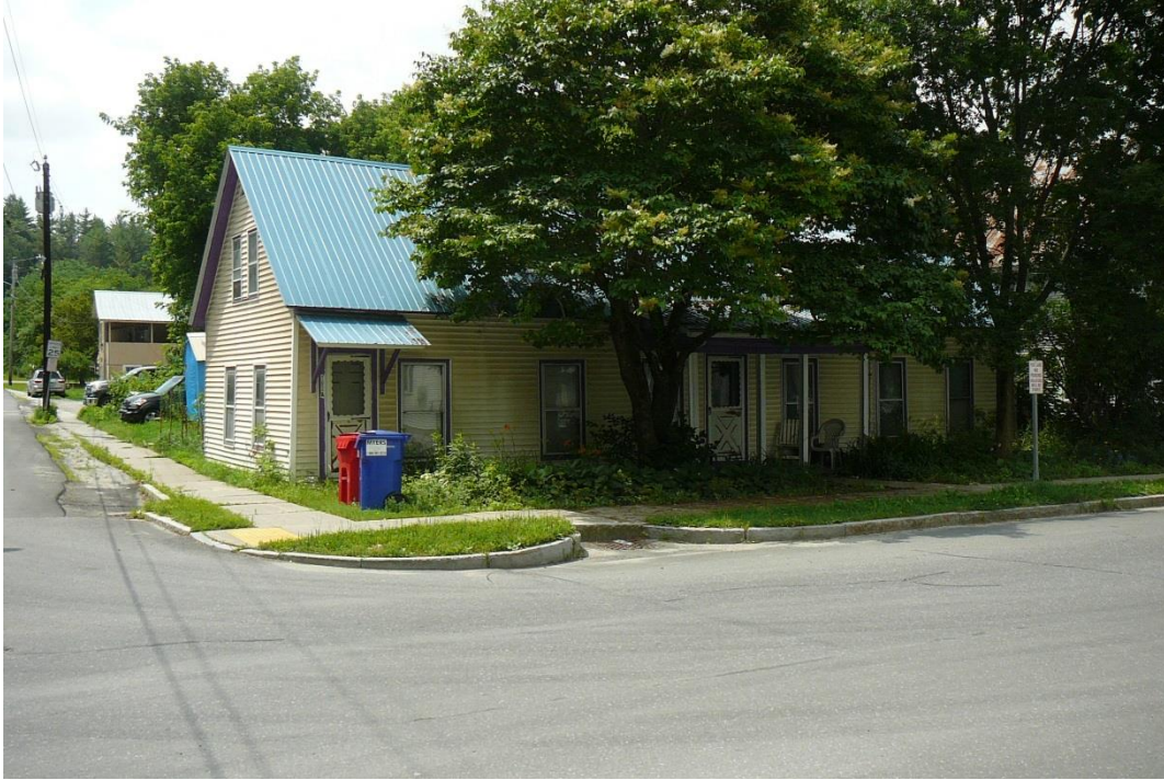
Figure 52. View southwest of 162 Main Street.
