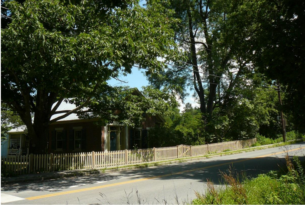
Figure 55. View northeast of 191 Main Street.
