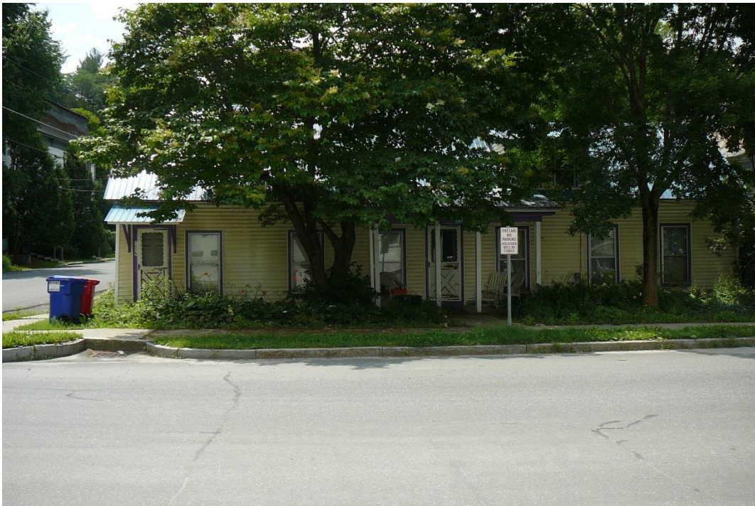
Figure 53. View south of 162 Main Street.
