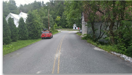
Image 4-1: Creamery Street Looking West
