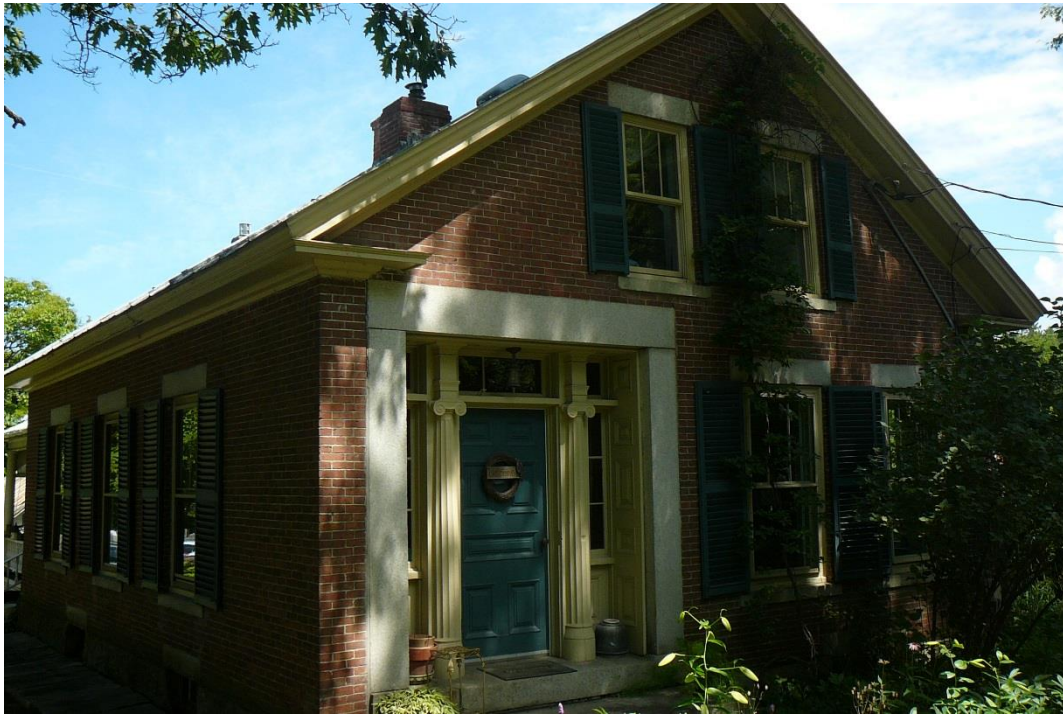
Figure 57. View northeast of 191 Main Street.
