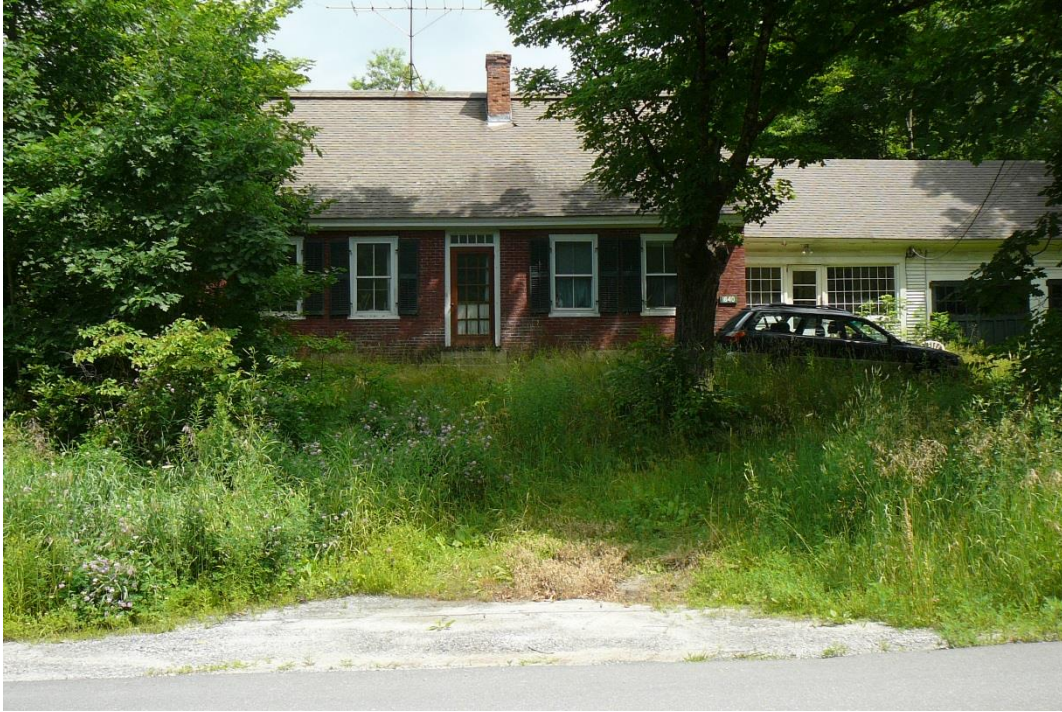
Figure 30. View north of 99 Brook Road.
