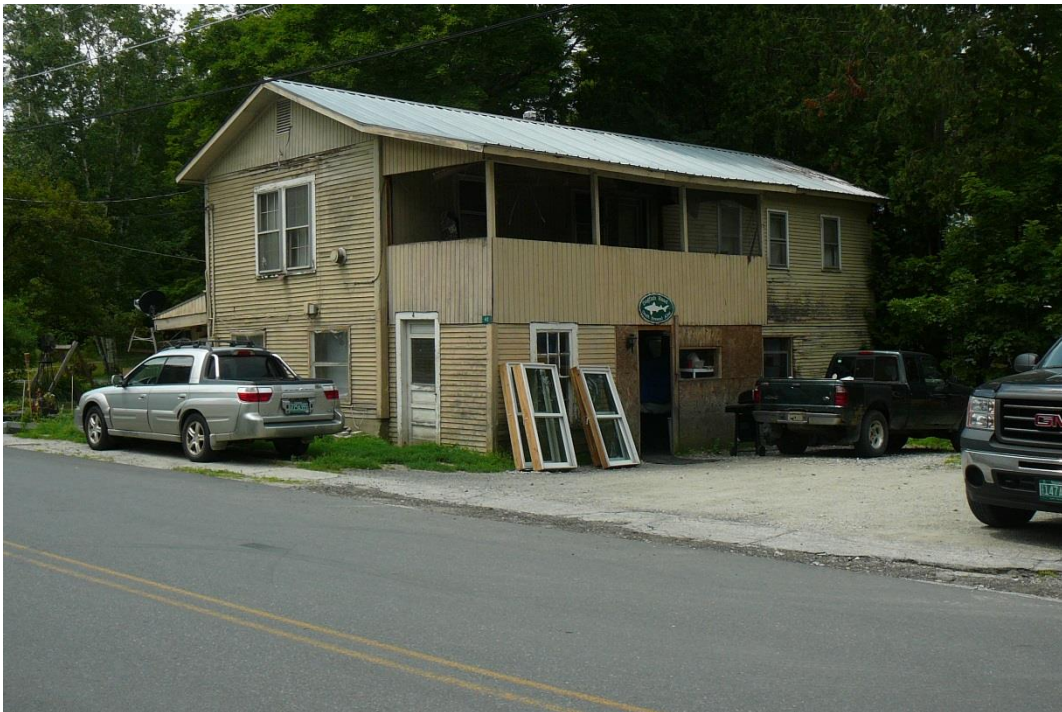
Figure 49. View southwest of 42 Creamery Street.
