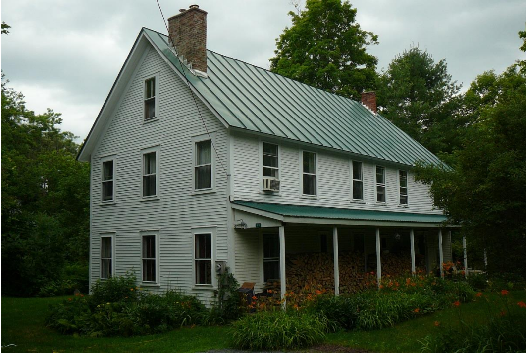
Figure 26. View northeast of 65 Brook Road.
