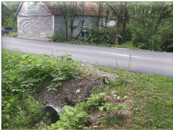
Image 4-5: Culvert and Historic Barn on Creamery Street.
