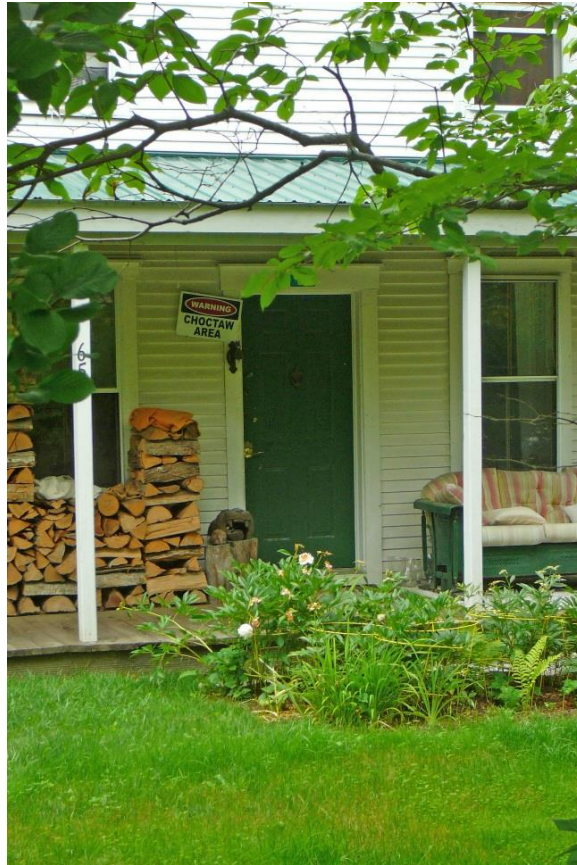
Figure 28. View northeast of front entrance door at 65 Brook Road.
