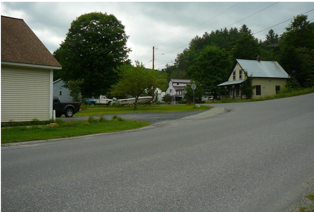
Figure 9. View southeast on Mill Street at the west end of the project area, with Brook Road stop sign at center; 133 Mill Street garage at left foreground.
