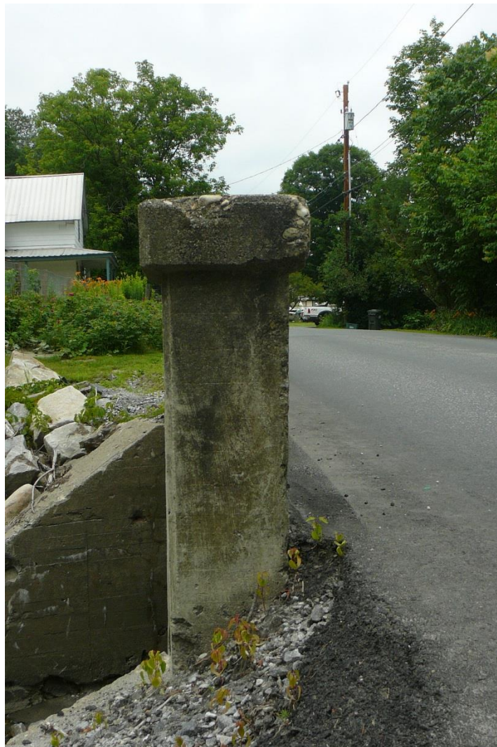
Figure 66. View west of Bridge 21 along Brook Road.
