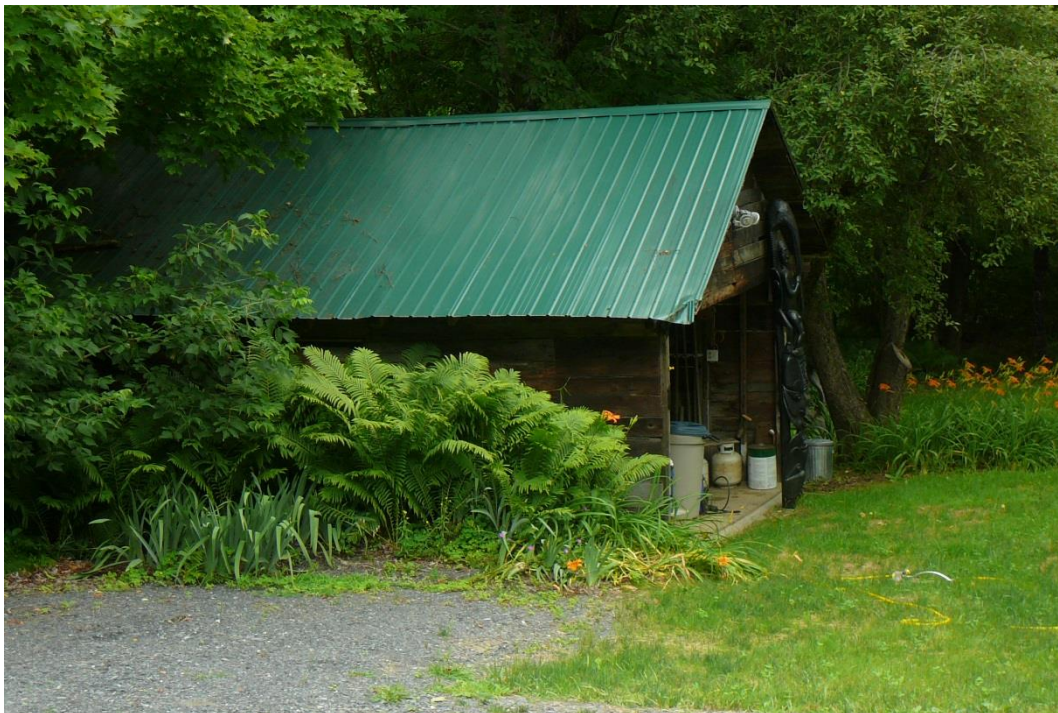
Figure 29. View northwest of garage at 65 Brook Road.
