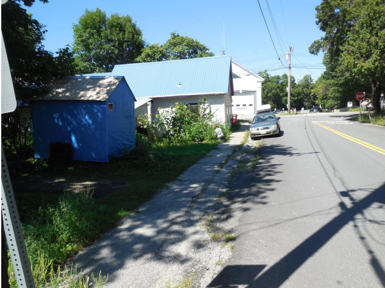
Figure 10. Photos looking north along Creamery Street towards the intersection with Main Street along the alignment of the proposed Plainfield STP BP15(16): Lower Village Sidewalk Project, Plainfield, Washington County, Vermont.
