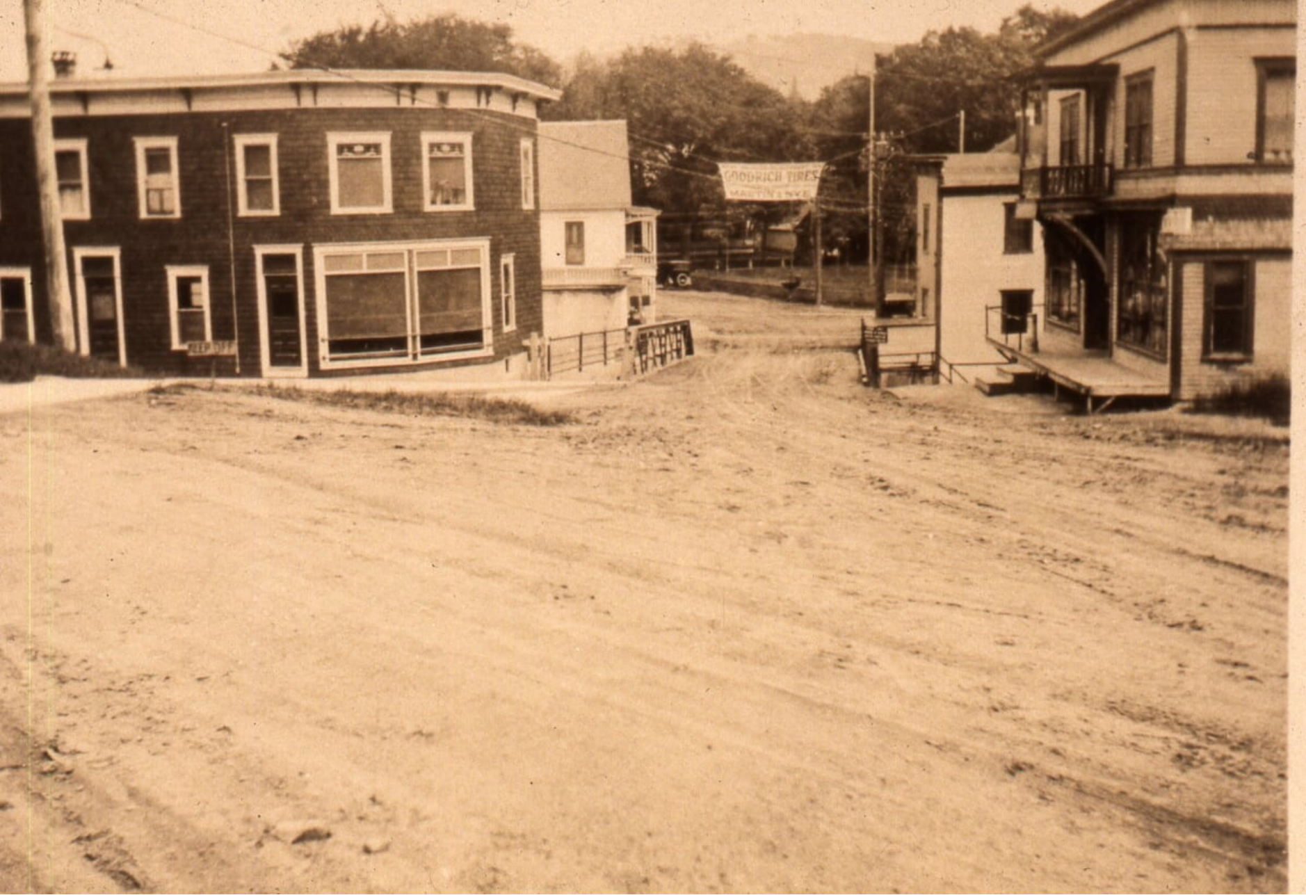
Martin Building on the left, built in 1919 Image provided by Susan Grimaldi, Plainfield Historical Society
