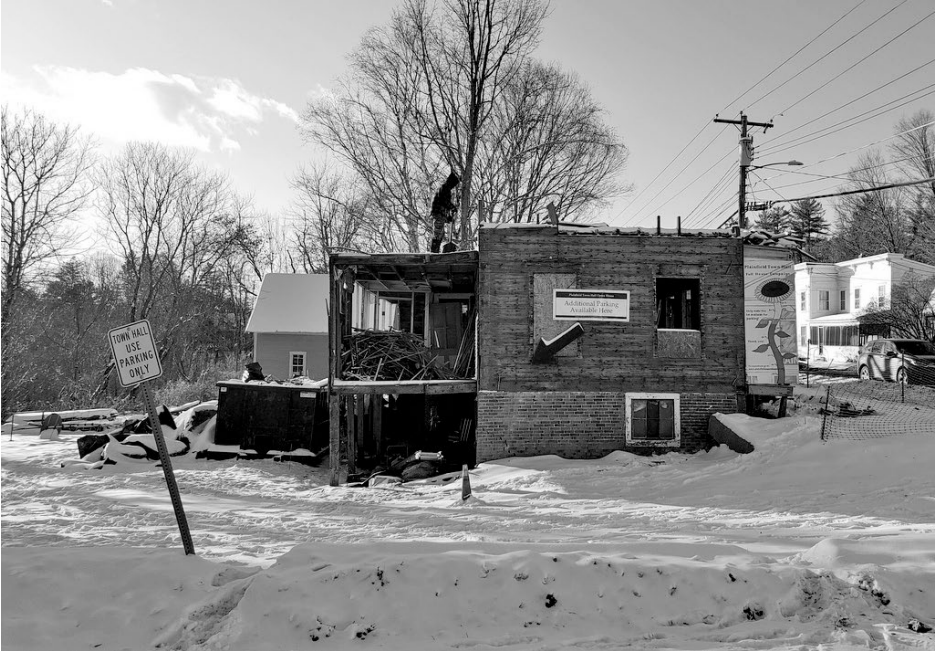
Ki Walker taking down the abandoned house at 25 High Street
