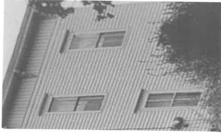
WEST HOUSE FACADE: FACING TOWARD RT WITH TREE COVER. THIS WILL BE A REPLICA OF THE EAST FACADE WITH CORBELS.
