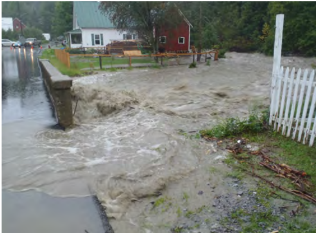
Figure 2. Upstream Face of the Brook Road Bridge at Full Flood Capacity (Source: Springston, 2011)
